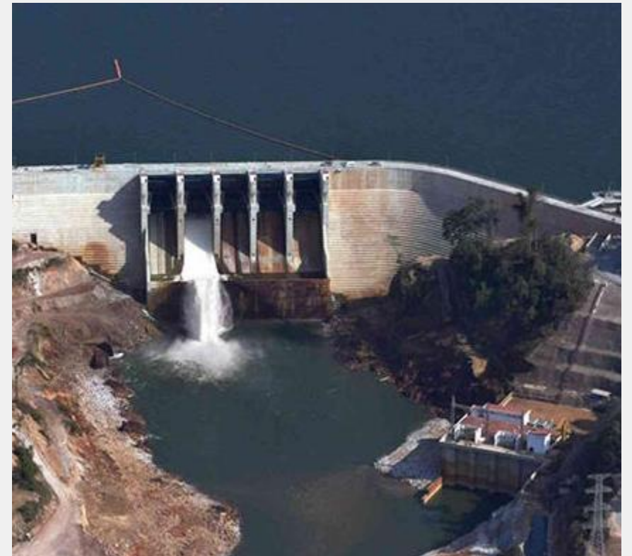
THPC 525 MW hydro power plant
