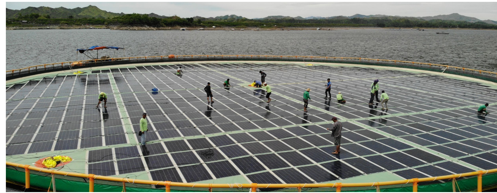
Pilot floating solar project, Magat
